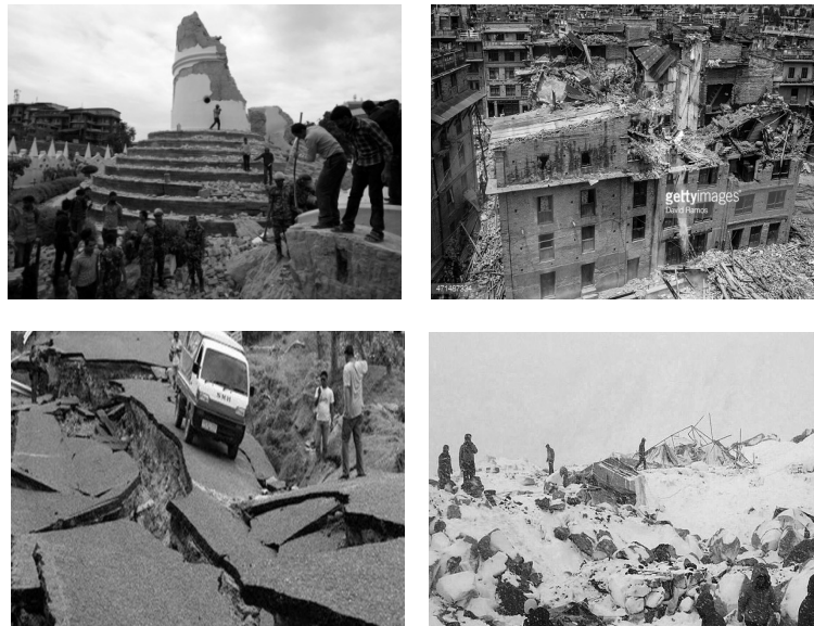
Figure 6: Different damages in Nepal during the earthquake (National Post News, globalnews.ca, mormonsoprano.com)
