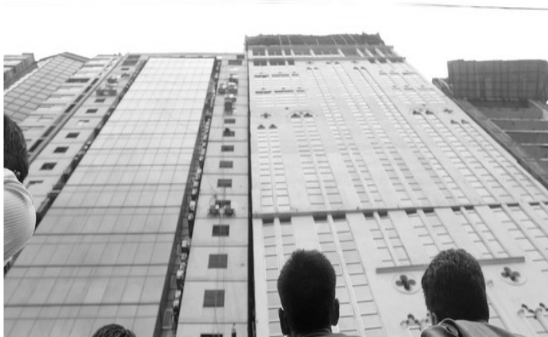
Figure 9: One building have tilted over another one (bdnews24)
