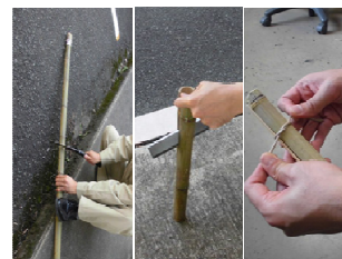
3) Cutting and tying bamboo bars
