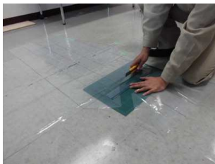
1) Drawing and cutting the sheet
