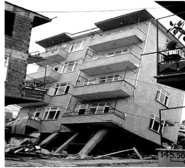
Collapse of building due to soft storey
