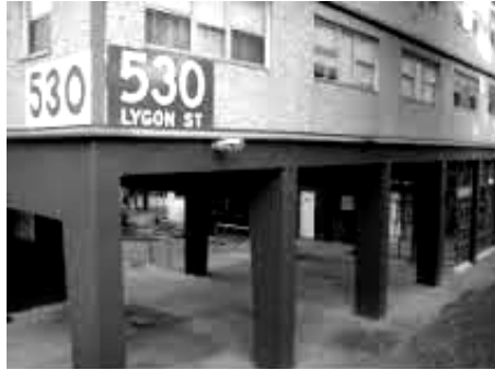
Building with soft Storey
