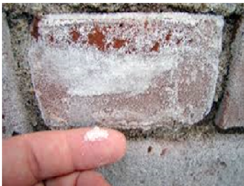
Figure 1: Effect of salinity of bricks and sands on masonry structures
