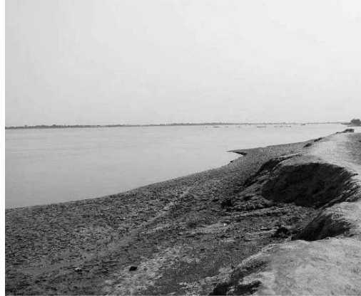
Figure 9: Canal bank erosion (Photo credit: Afjal Hossain)
