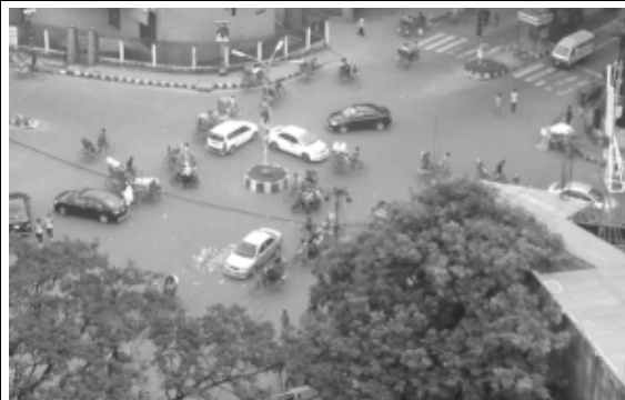
Figure 4: Absence of Channelization
