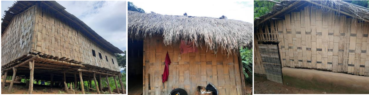
Figure 6: The mat used at outer façade and the thatch roof (Captured by author, October 2021).
