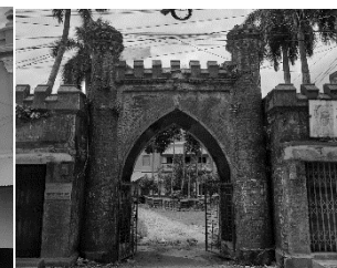
Fig 7: Gateway of DewanBari
