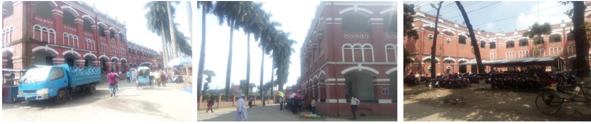
Figure 02: Jashore Collectorate Building (Source: author constructed)
