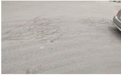
Figure 11 : Fatigue Cracking
