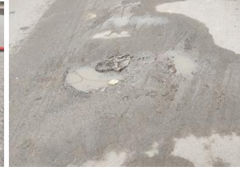
Figure 13: Potholes
