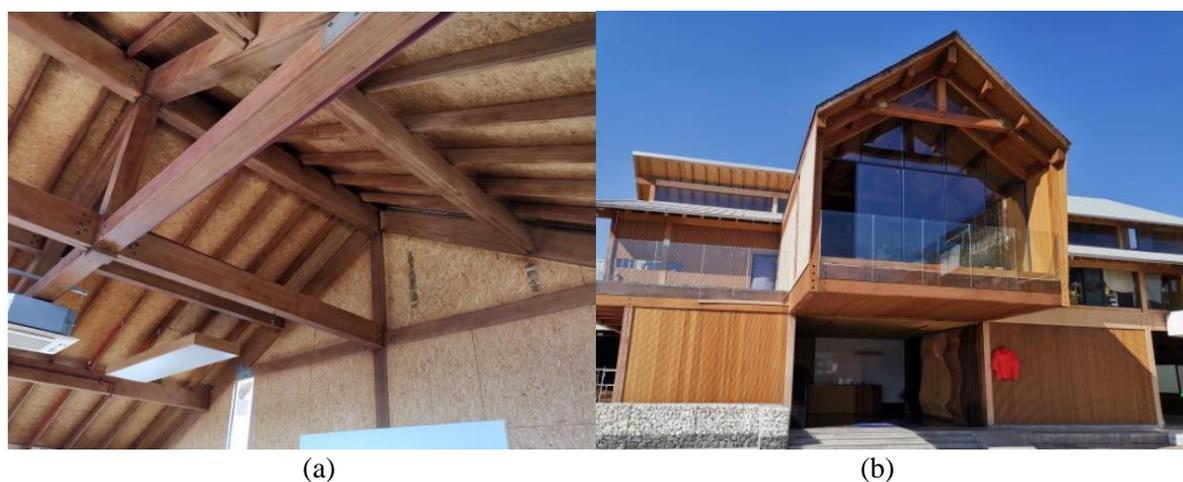
Figure 3: Three – storied office building constructed using LBL members (a) structural system of the roof and (b) front view (Photo courtesy: Su et al. (2021) )
