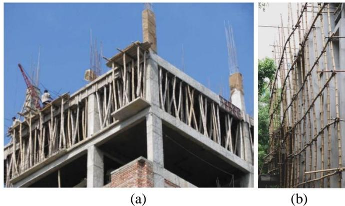
Figure 10: Bamboo poles used for construction (a) propping (Mukul & Rana, 2013) and (b) temporary formworks (Riyad, 2023)
