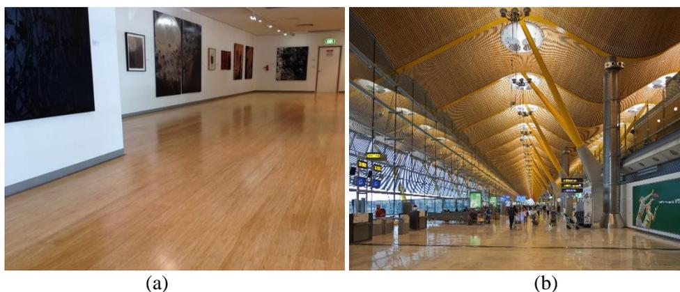
Figure 2: Application of bamboo panels (a) flooring (Flooring, 2023) and (b) ceiling of Bajasas International Airport, Madrid, Spain (Wikipedia, 2013)
