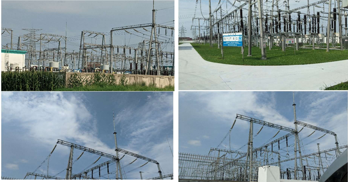
Figure 1: Photo captured during site inspection
