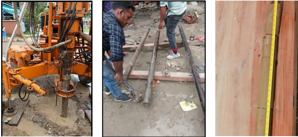
Figure 6: Core sample collection using core drill and sampling method
