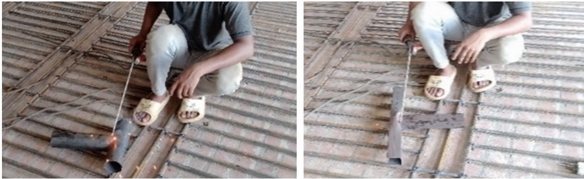
Figure 2: Welding steel tubular section to build T-joints
