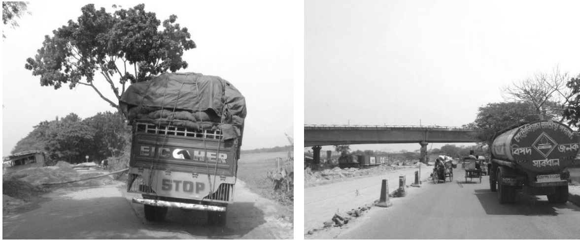
Figure 3: Typical scenarios of absence of advance warning signs at work zones in Bangladesh
