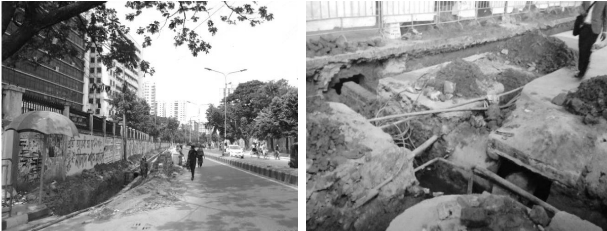
Figure 6: Common scenarios of absence of pedestrian facilities at work zones
