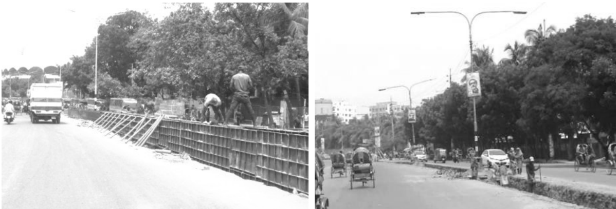
Figure 7: Common scenarios of negligence of safety by workers at work zones in Bangladesh
