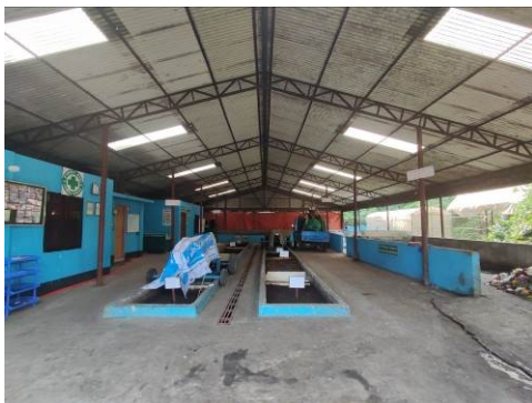
Inside view of the plant
