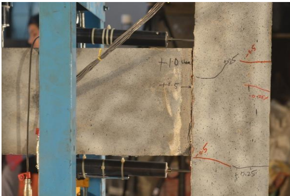
Fig. 4.7: Failure Mode of Specimen-3
