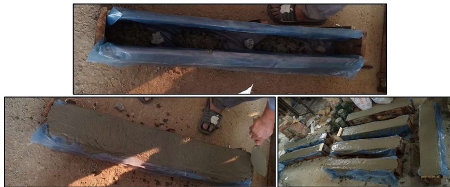
Figure 2: Casting of Beams
