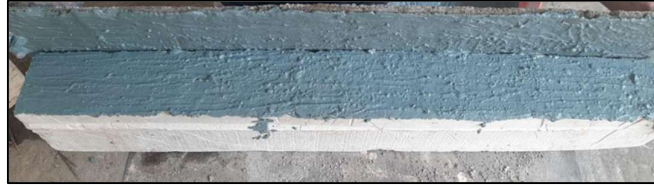
Figure 6: Retrofitting Using Epoxy Resin
