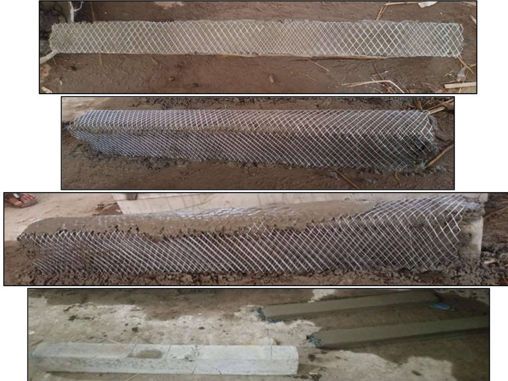
Figure 7: Orientation of Wire Mesh and Retrofitting Process
