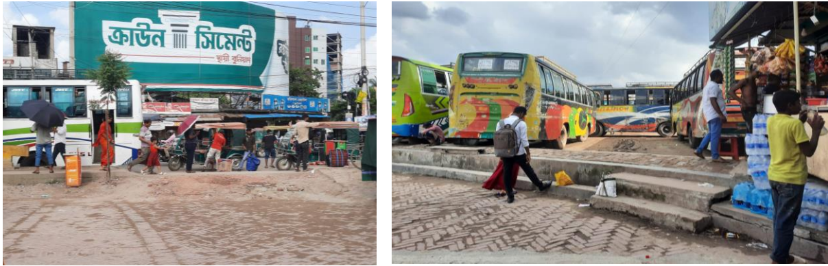
Figure 5: Entry of the terminal building blocked by mounted earth (Left), Walkway ends at the front of a shop (Right)
