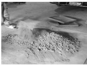
Figure 2: Concrete Dry mixing
