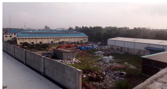
Figure 4: Lack of proper waste management system
