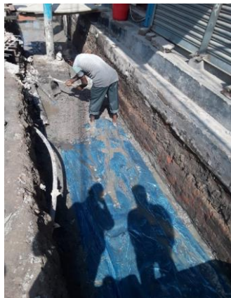
Figure 2(b): CC casting of drain bed is on progress at site.
