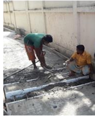
Figure 4 (c): RCC casting of drain top removable slab is ongoing
