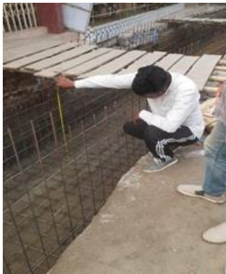
Figure 3 (a): Rebar binding is being inspected at site.
