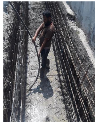
Figure 2 (c): RCC drain base casting is ongoing at site.
