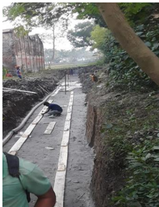
Figure 2 (a): Wooden formworks are being prepared for drain bed casting.
