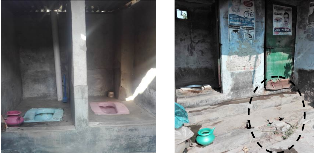
Figure 3: Two unit toilet, Rupsha slum
