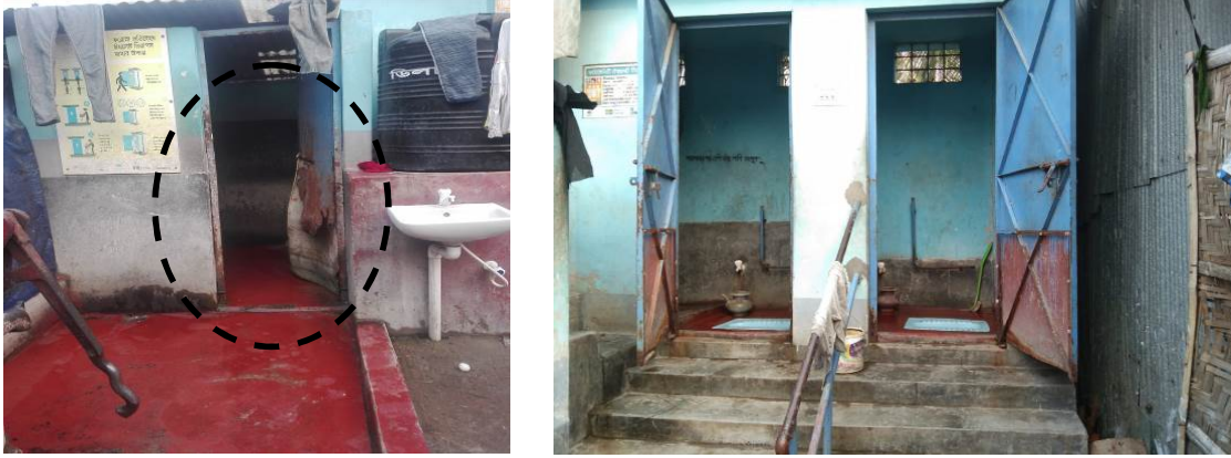
Figure 5: Two unit toilets with bathing, Greenland Abashon slum
