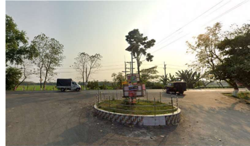
Figure 12: Risky Access to Highway
