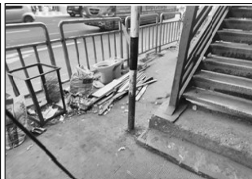
Figure 18. Dirt right beside the stair case.
