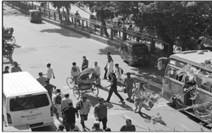
Figure 20. Series of guardrails being missing along the roads.
