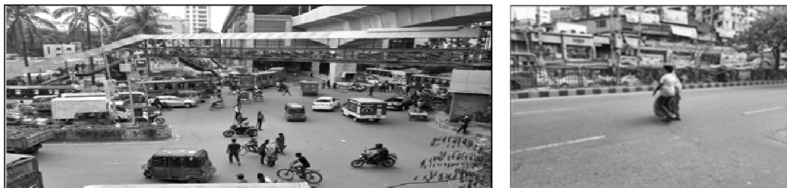
Figure 6: People are crossing by the road underneath footover bridge
