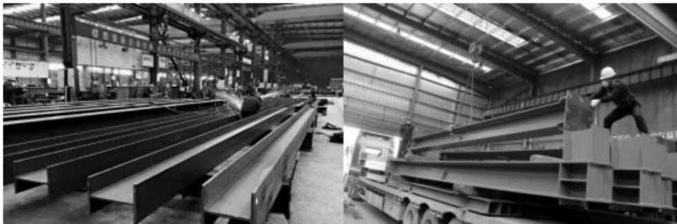
Figure 7: It only took 40 hours for a steel structure manufacturer from Anhui Province to load and deliver 2,000 sets of standard steel structural components to the Leishenshan Hospital location (Wen-tao et al., 2020).
