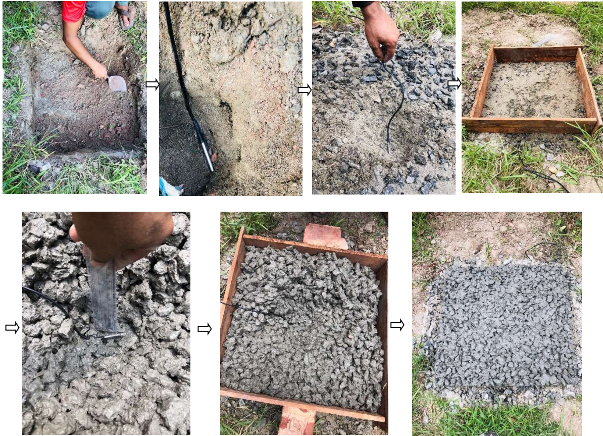
Figure 2: Construction and sensor inserting
